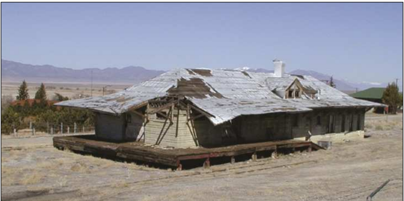
This was the condition of the building when the project started.
