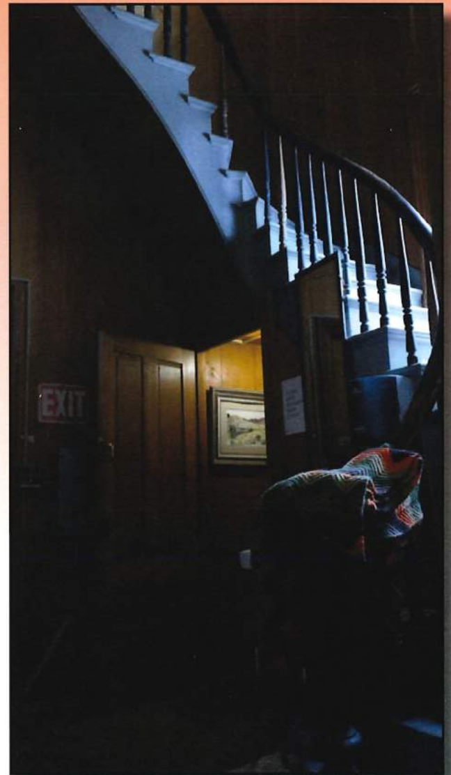
Figure 3.39 South wall of Stair 3.
