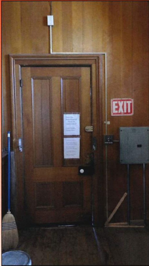
Figure 3.38 Door to exterior on east wall of Stair 3.
