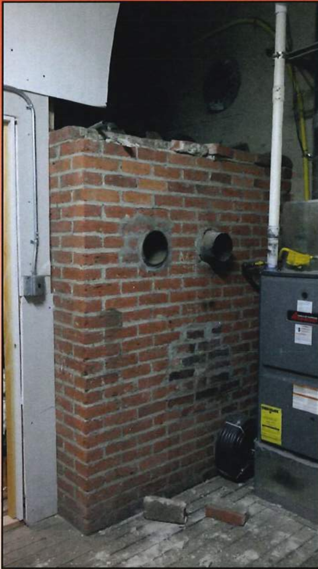
Figure 3.17 South elevation of historic brick furnace in Mechanical Room.
