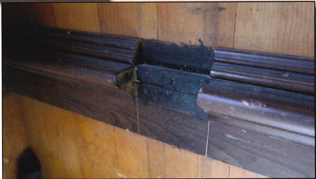
Figure 3.48 Missing piece of chair rail on north wall of Vestibule historically accommodated organ equipment.
