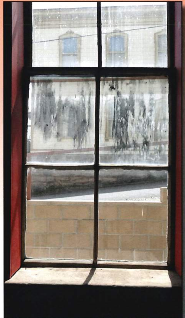
Figure 3.24 Oxidized film on window in Infant Classroom/Exhibit Hall.
