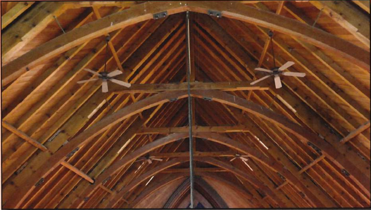
Figure 3.52 Open trusswork of the Nave.
