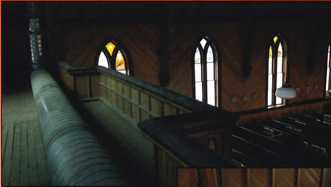
Figure 3.74 Gallery looking northeast.
