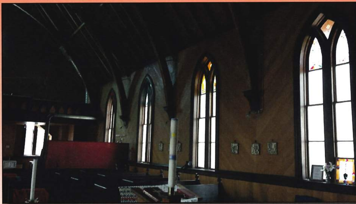
Figure 3.54 Truss-window pattern along north wall of Nave.
