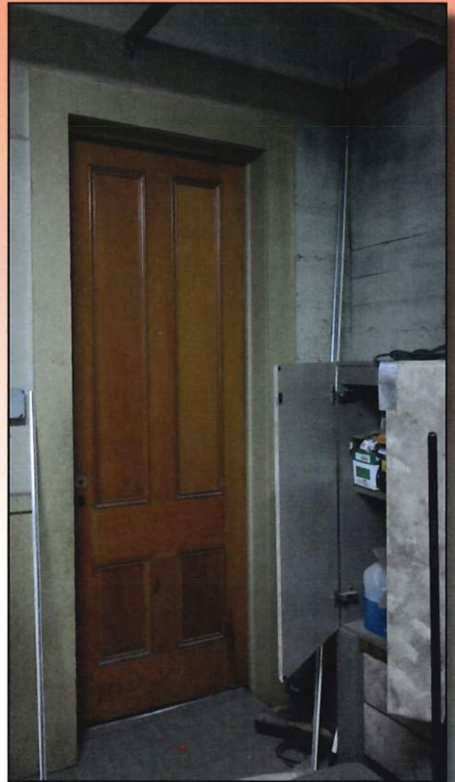
Figure 3.18 Varnished pine door leading from Mechanical Room to Infant Classroom/ Exhibit Hall.
