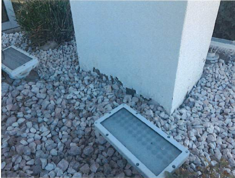
Photos of damage to the pillars of the La Concha:
