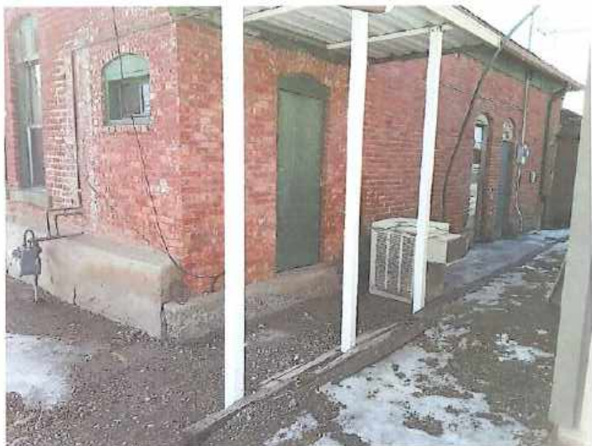
North Side (Rear) of Building Facing West
