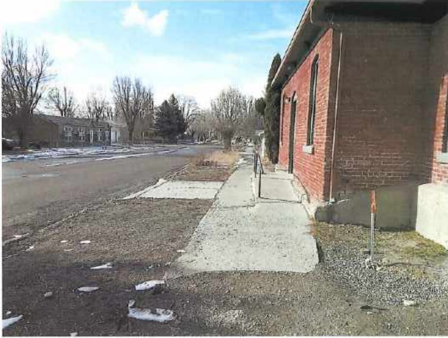
Front of Building Facing West
