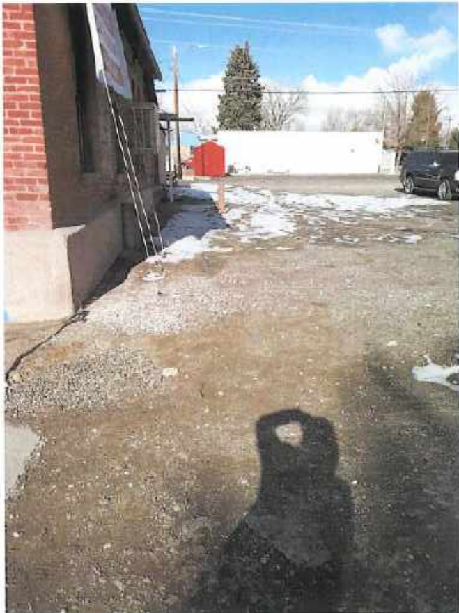
East Side of Building Facing North
