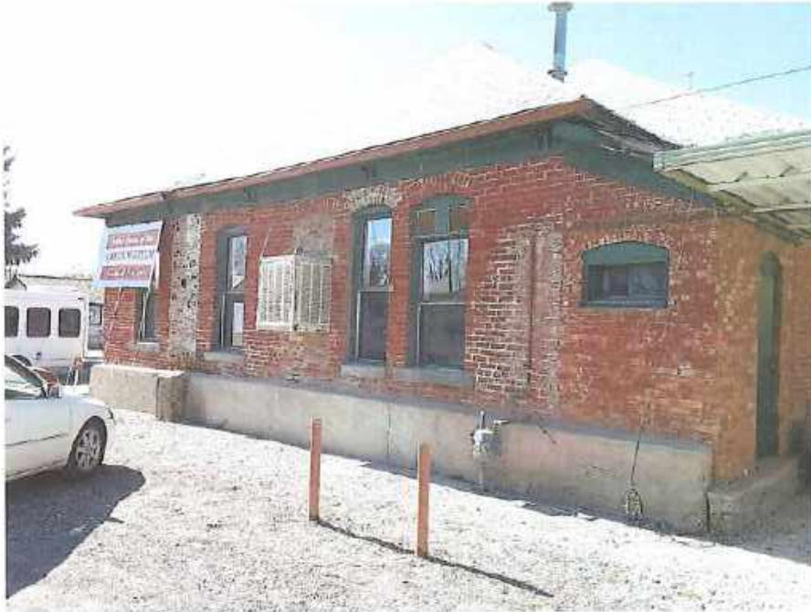
East Side of Building Facing West
