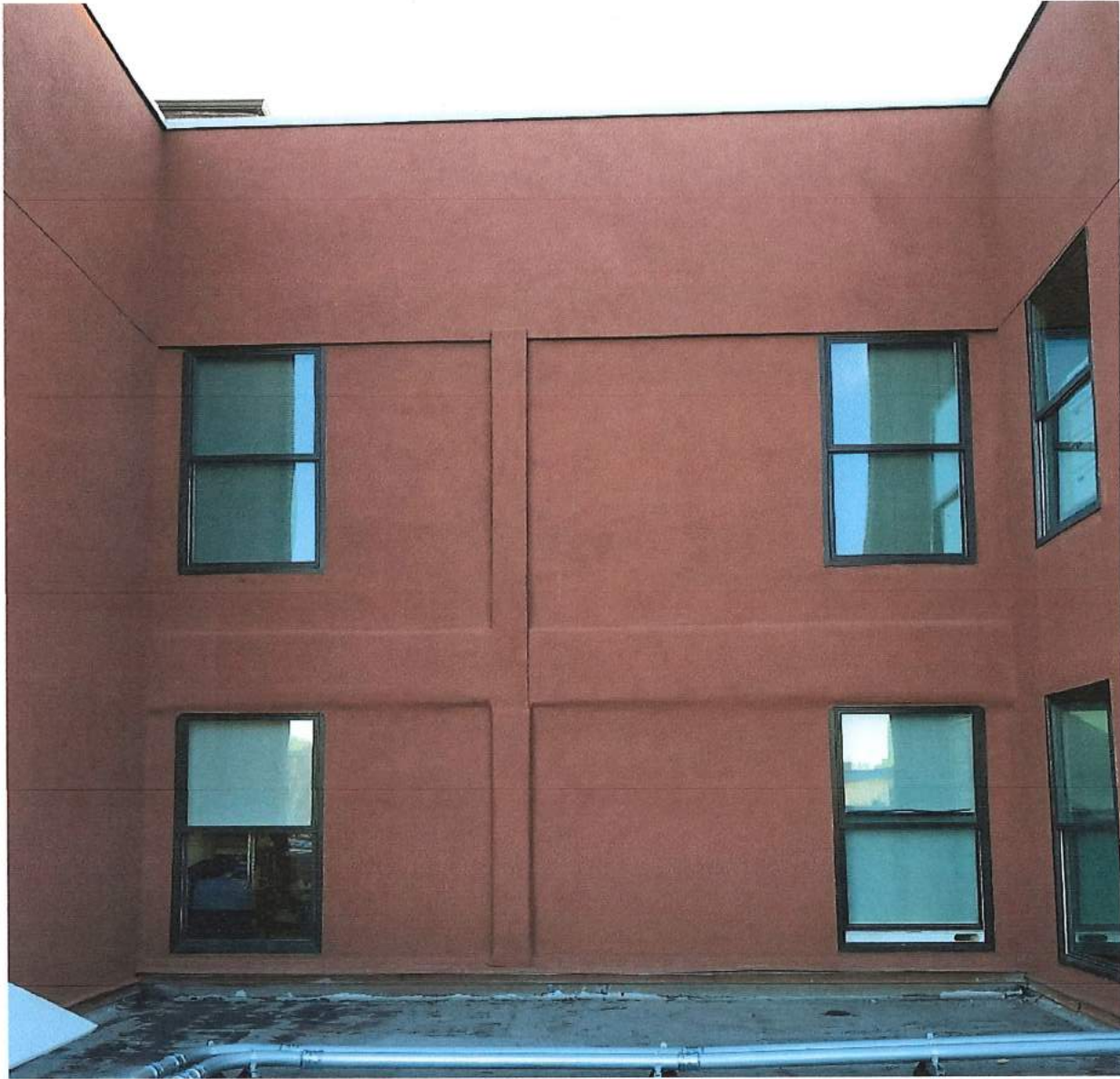
Photograph depicting the completed stucco replacement in Phase 13 of the Pioneer Hotel renovation project, partially funded by the CCCHP (2016-2017 grant year). Work completed by L&C Plastering. On the site plan found in the CentiMark proposal, this is the boundary between Sections 2 and 4.
