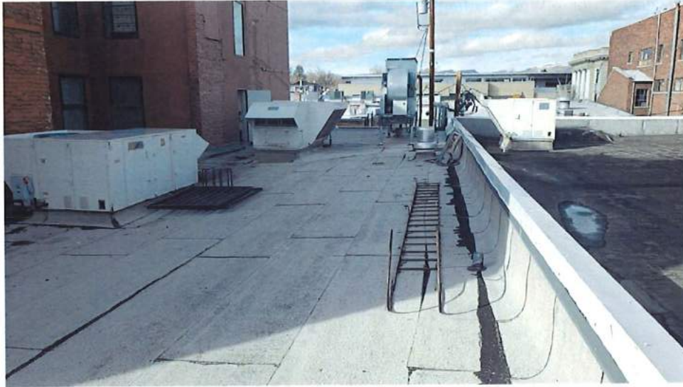
Section: Section 2 Area: Overview Caption: The Existing Metal Counter-Flashing Will be Replaced with New During the Re-Roof Process
