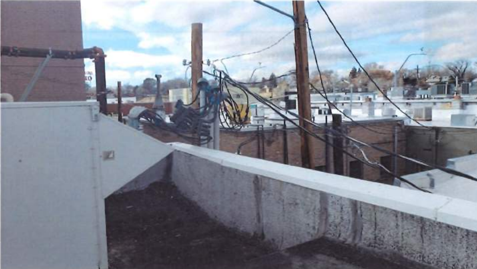
Existing Safety Condition
