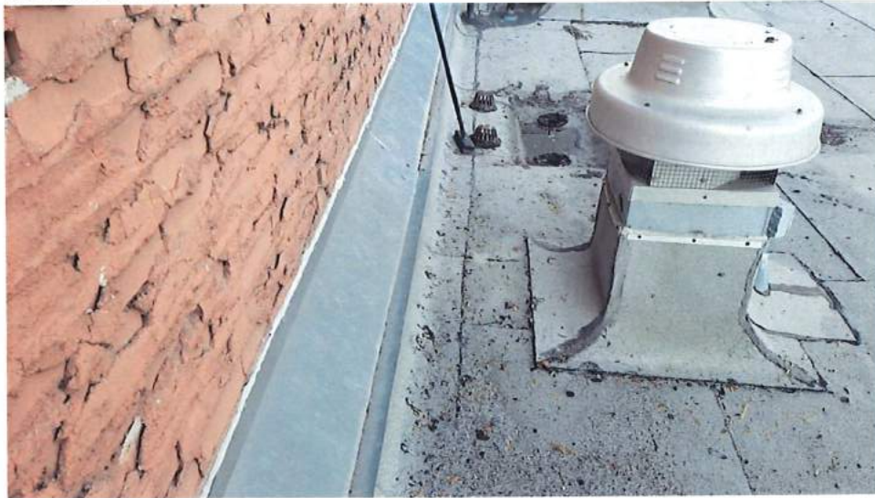
Section: Section 2 Area: Overview Caption: The Existing Metal Counter-Flashing Will be Replaced with New During the Re-Roof Process
