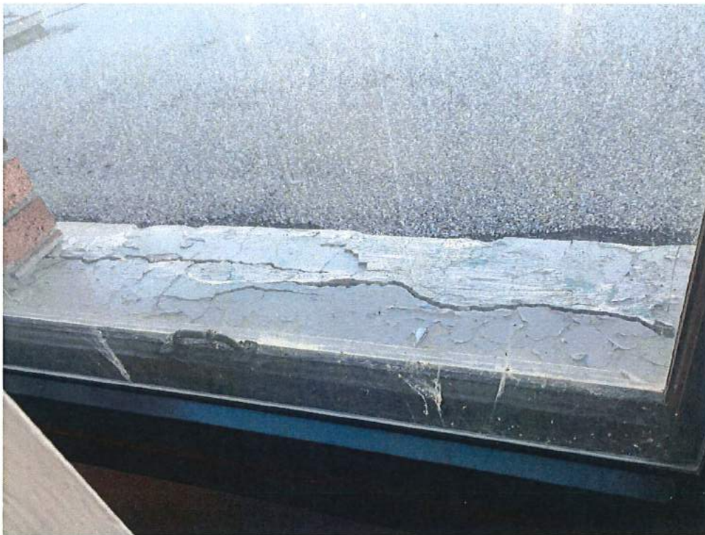
Cast stone window sill on North side of building.
