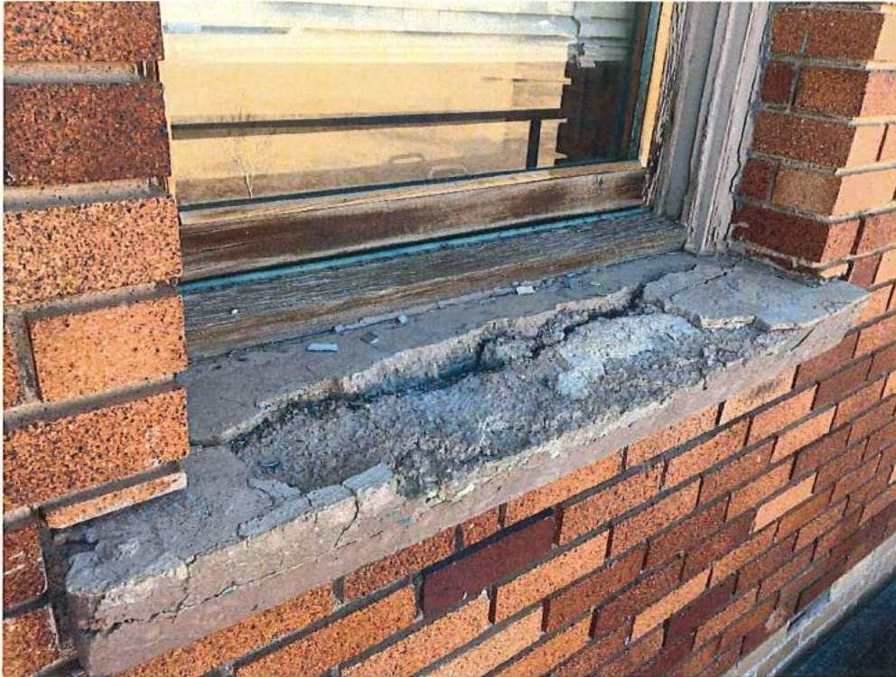
Cast stone window seal and deteriorating sash and frame on the west side of building.
