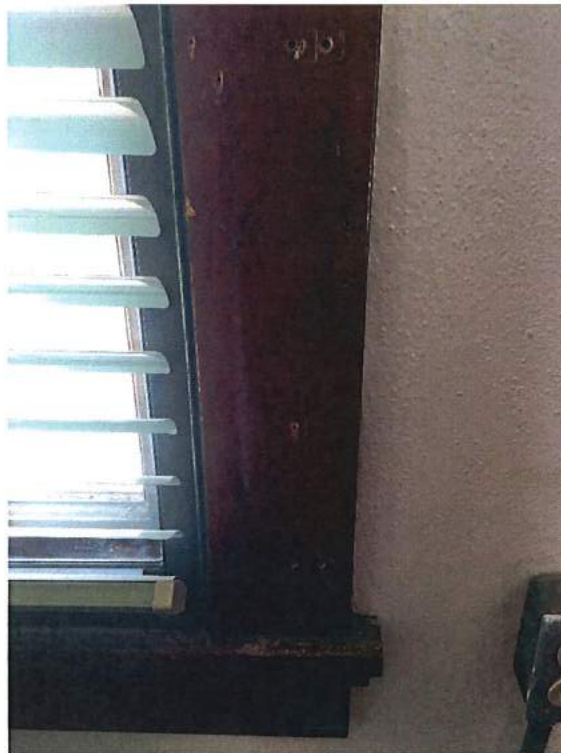
Interior of window on the East of the building showing damage from carelessly installed accessories over the years and water damage along bottom of frame.
