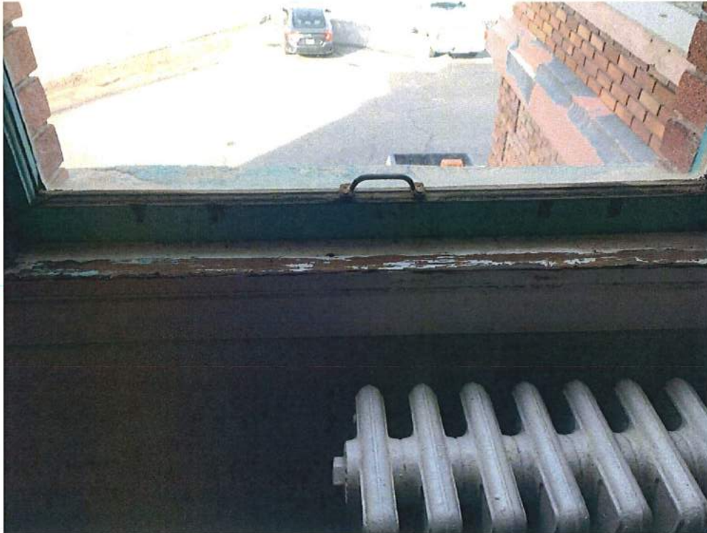
Interior of window on East side of building showing damage due to water infiltration and damage caused by interior storm windows that are believed to installed in the late 80's.
