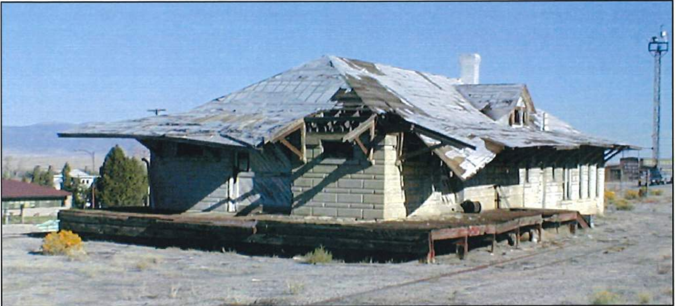
Southeast Corner of the Depot at the beginning of the project.
