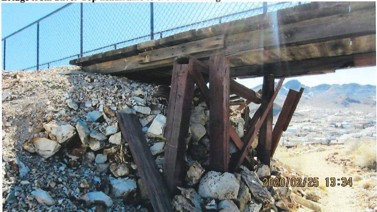
Bridge from Silver Top headframe to orehouse facing south.
