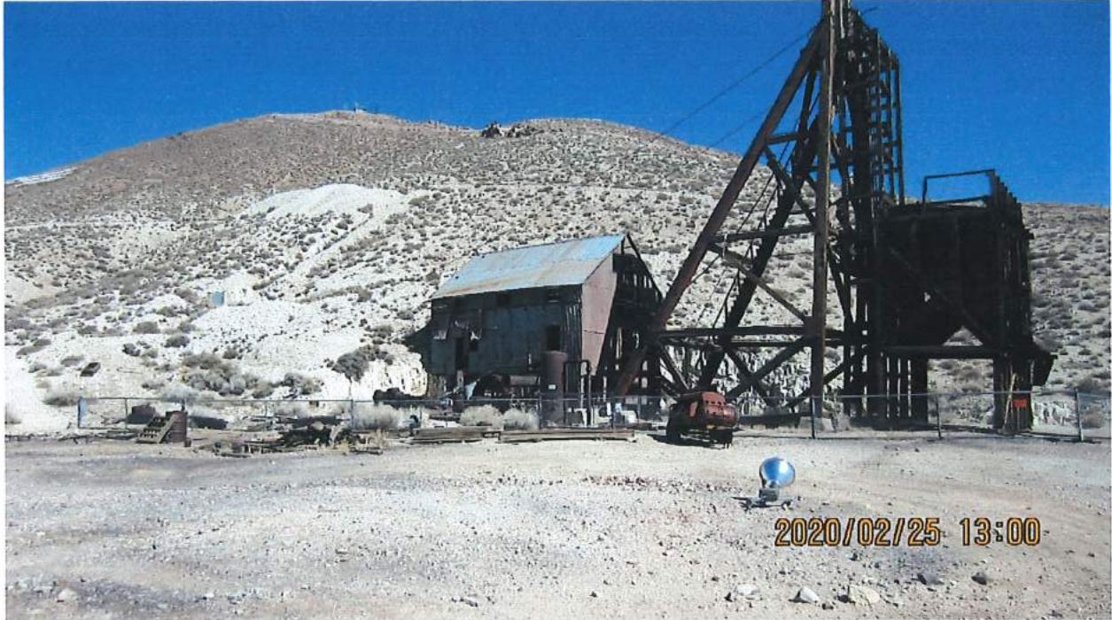
Desert Queen headframe and hoist house facing northeast.
