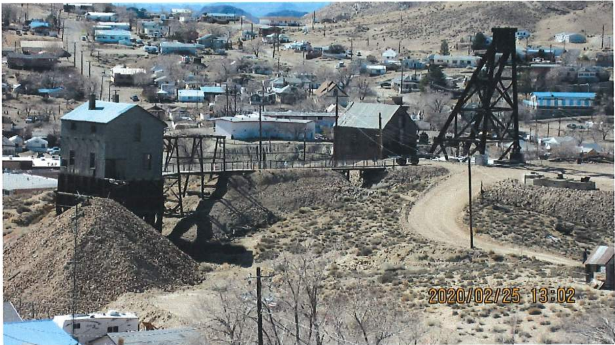
Silver Top headframe, hoist house, bridge & trestle, and orehouse facing southwest.
