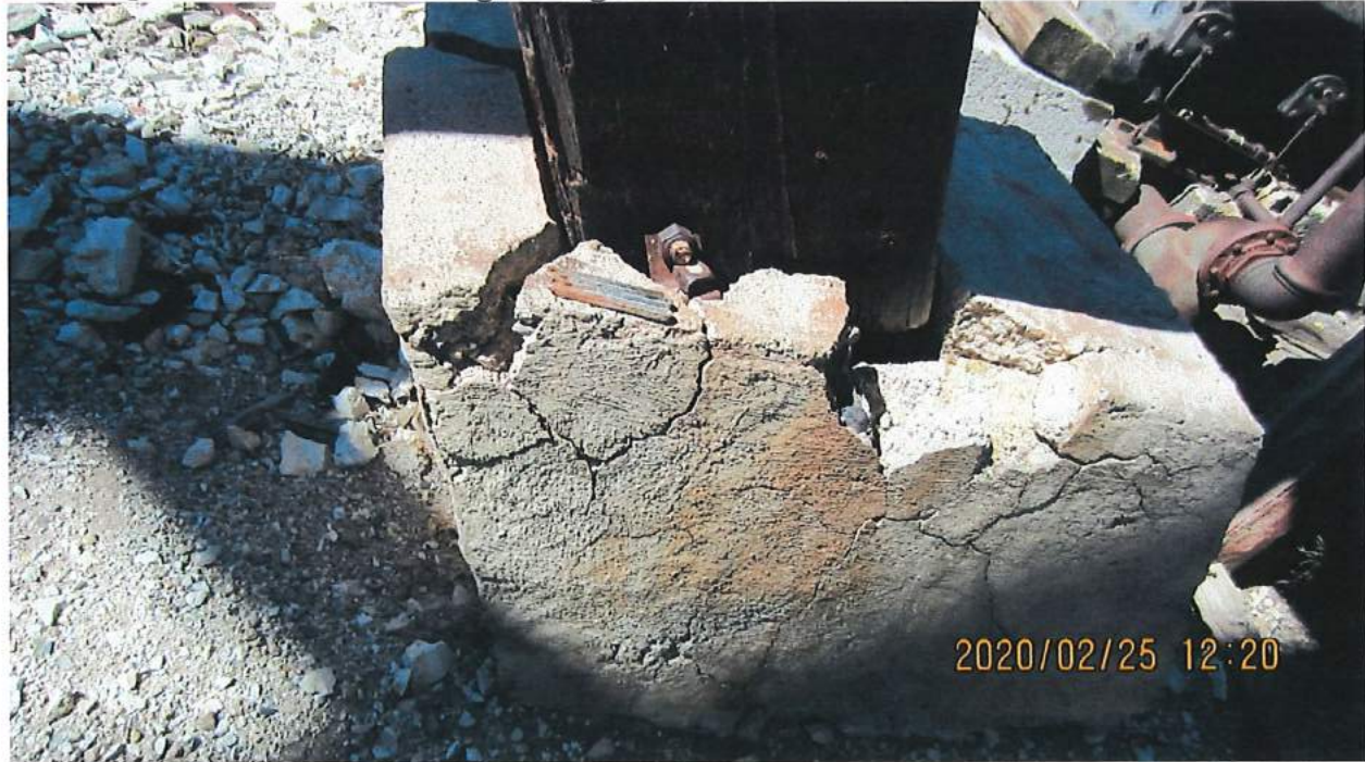
Desert Queen headframe footings facing southwest.
