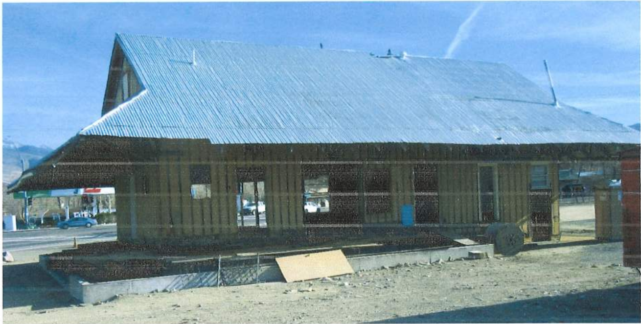
Fig. 6 – Elevation from NW, track side. (Note that it is hard to get a good picture due to our narrow-gauge boxcar as well as stored rail being on this side next to Gold Creek.)
