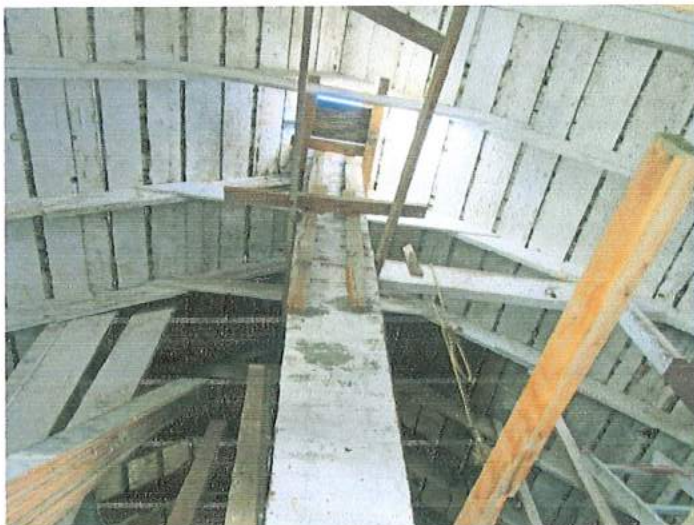
Fig. 13 – Inside freight room, looking NE from door from passenger room. The floor is original rough-cut lumber. The inside of the boards of the board-and-batt construction are rough, and were painted boxcar red. The door and window opening at the Keeler end (far wall) were resident-added and will be repaired. There are significant openings on the sides where the freight doors once were and also where residents added a bedroom (on back right). We salvaged portions of the original freight doors, which residents used to fill in openings. The 2"x4" rafters were resident-added to create a ceiling. They will be removed.
