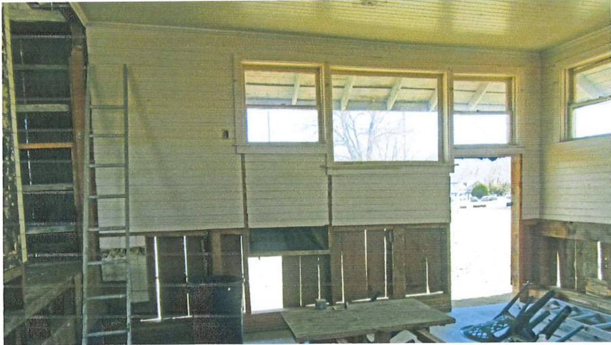
Fig. 11 – Inside passenger waiting room looking toward the SW, non-track side. Note the original door opening on the far right. There is a resident-added window to its left and a window in the upper portion of an original window farther left. On the lower wall behind the modern ladder is the outline of the original steep stairs up from the passenger room to the freight room (which is to the left). The walls and ceiling still have much of the original bead-board.
