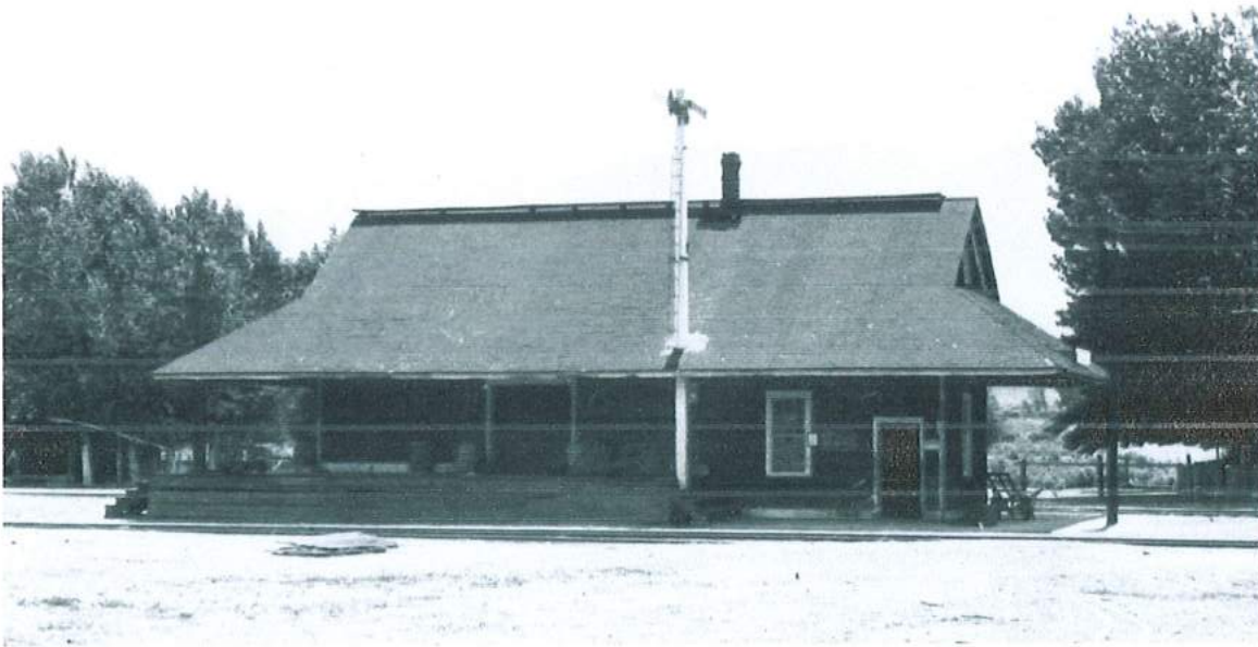
Fig. 7 – Depot from track side in 1907. SP added the train order board (white post) but other than that had changed the depot very little by this time. This is roughly the same view of the depot as in shown before deconstruction of resident-added rooms in Fig. 1.
