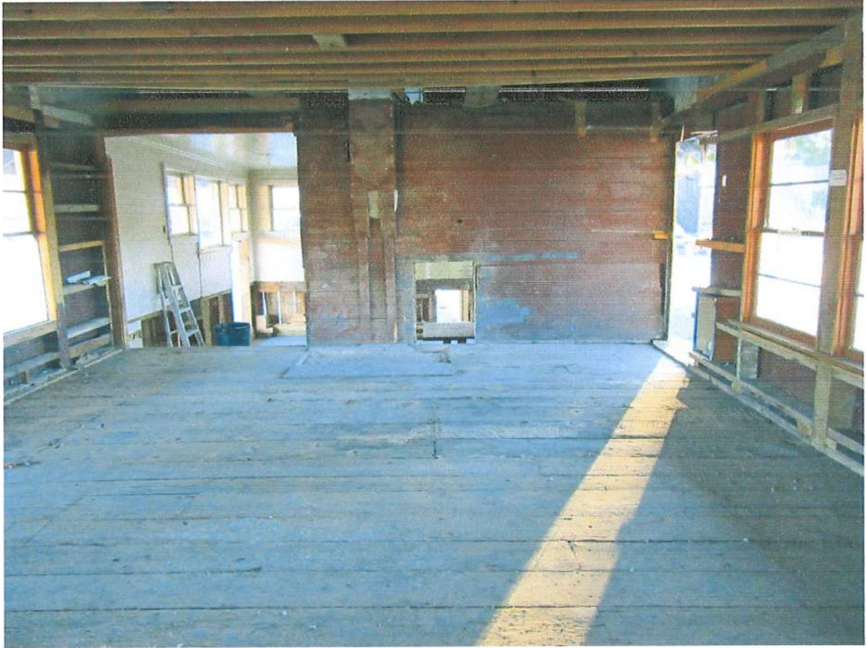
Fig. 15 – Inside freight room, looking SW toward passenger room. Rough-cut boards, painted boxcar red, are still in place on walls. On the outside walls these are milled flat on the outside.
