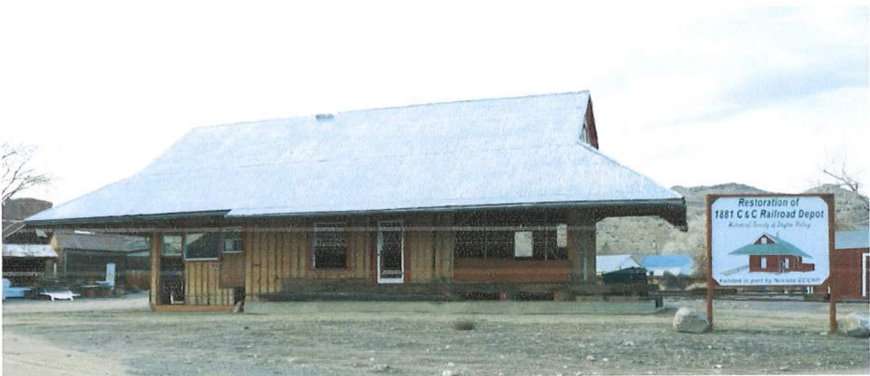
Fig. 3 – Depot in new location viewed from SE (near corner)
