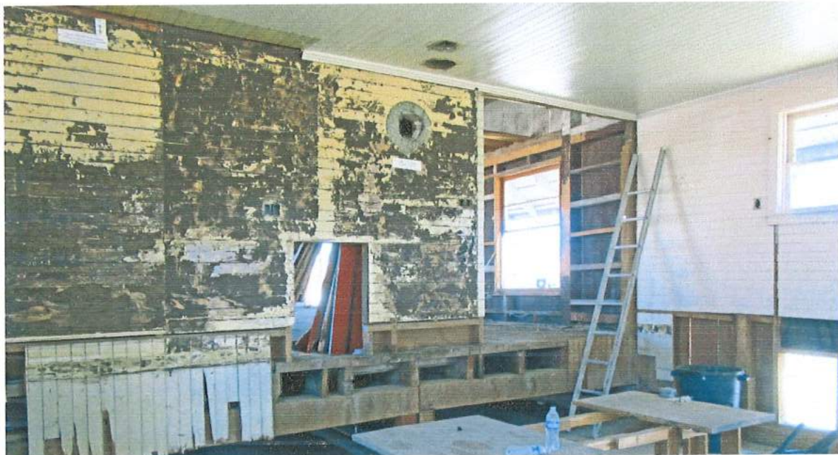
Fig. 12 – Inside passenger waiting room looking toward the ENE into the freight room. Originally there was a door across the opening to the right. The wall between the rooms has been damaged by resident-added tile but shows some evidence of scorching prior to be used as a residence. There is also an opening (near the center of the photo) where the agent passed items into the freight room for weighing. The opening for the potbelly stove is on the upper wall.
