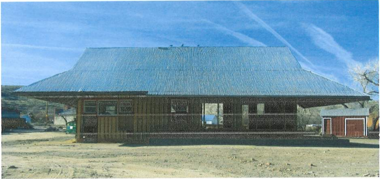
Fig. 4 – Elevation from SE, non-track side. The passenger depot is to the left, the freight room to the right (including missing freight doors). The Section Shed is shown past the depot on the far right.
