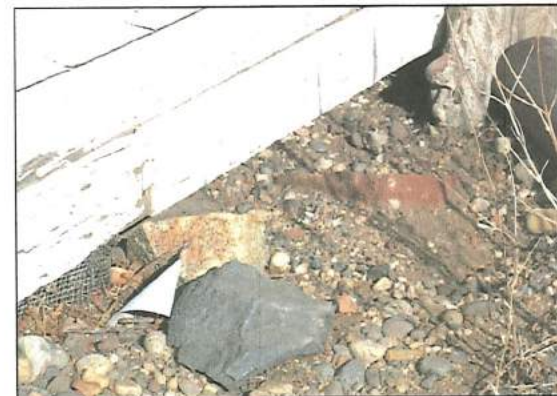
Holes in the house foundation where original granite rock foundations have deteriorated, at points HV-2, HV-3 and HV-4.
