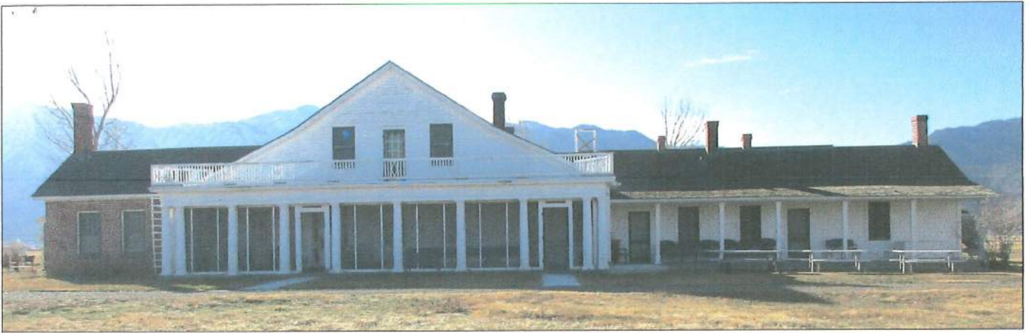
H-2: View from east
