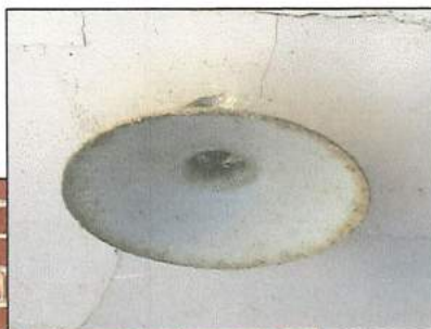
Above and below: Deteriorated and dangerous electrical light fixture (CV-5) and switch (CV-6).
