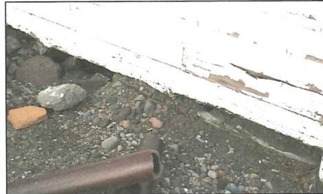
Holes in the house foundation where original granite rock foundations have deteriorated, at points HV-2, HV-3 and HV-4.
