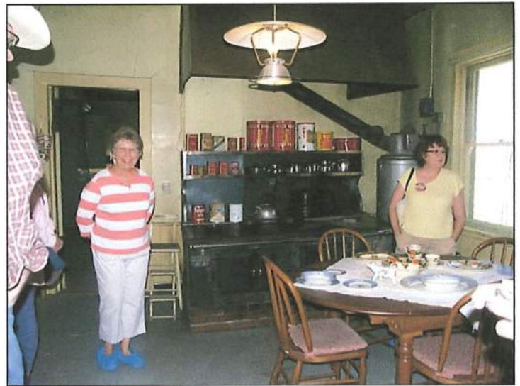
Tour group. Problematic foundation damage is evidenced by cracks in chimney wall.
