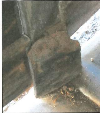
Left: Deteriorating and damaged trim (GV-6) and electrical (GV-2).
