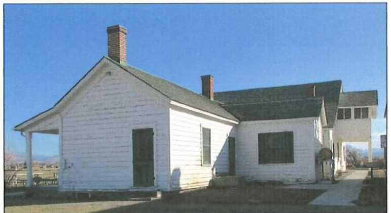
H-1: View from north Oblique view to also show a portion of west elevation.
