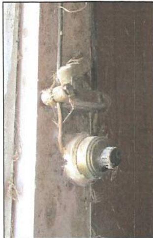
Above and below: Deteriorated and dangerous electrical light fixture (CV-5) and switch (CV-6).
