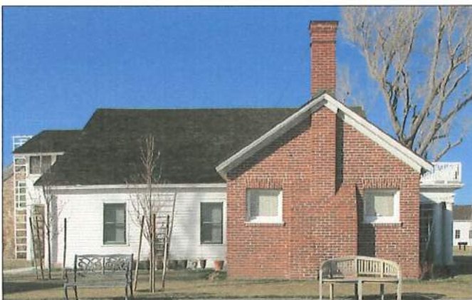
H3: View from south Brick walls repaired Summer 2019.
