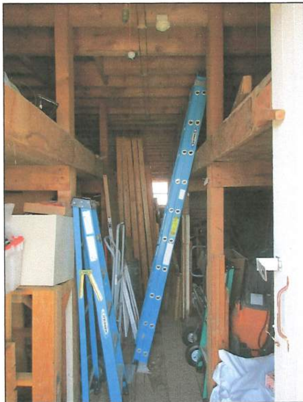
Interior view of south room from CV-2.
