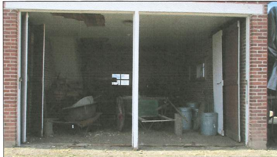
View inside with both doors open from CV-1.
