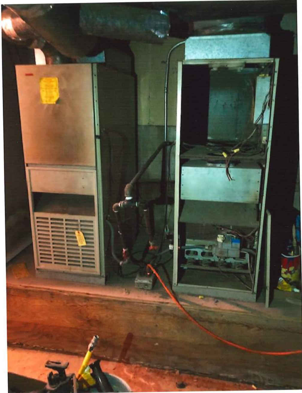
PICTURE #3 OLD HEATING SYSTEM IN THE CELLAR
