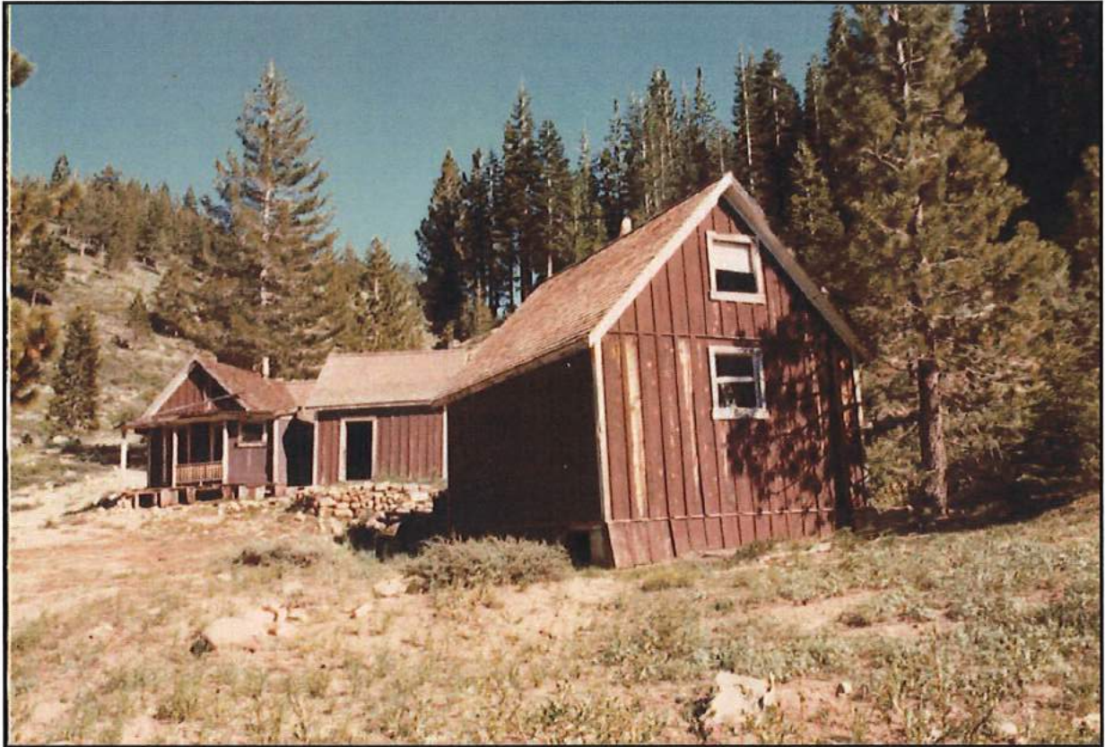
Site Picture with Bunkhouse in the Foreground – early 1980's before collapse
