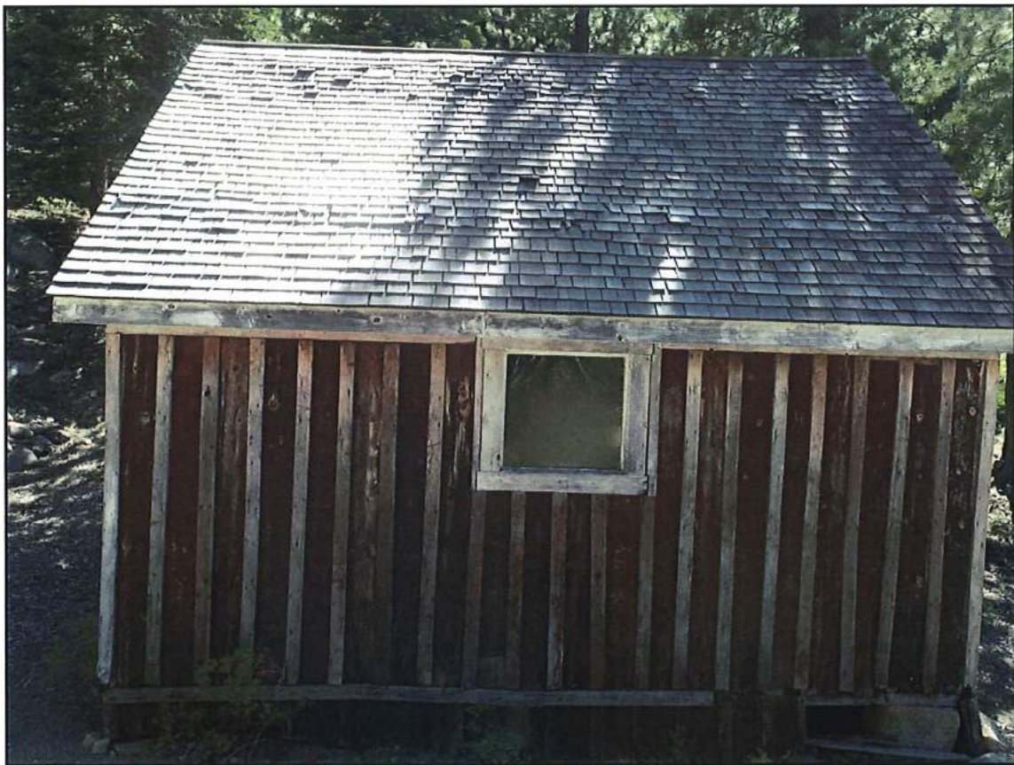
North Side of Structure (looking southwest)
