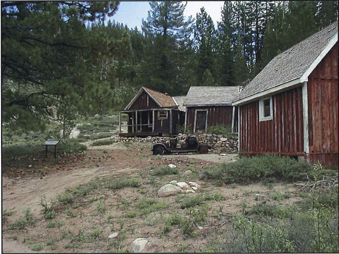
Site Picture with Bunkhouse in the Foreground (early 2000's looking northeast)
