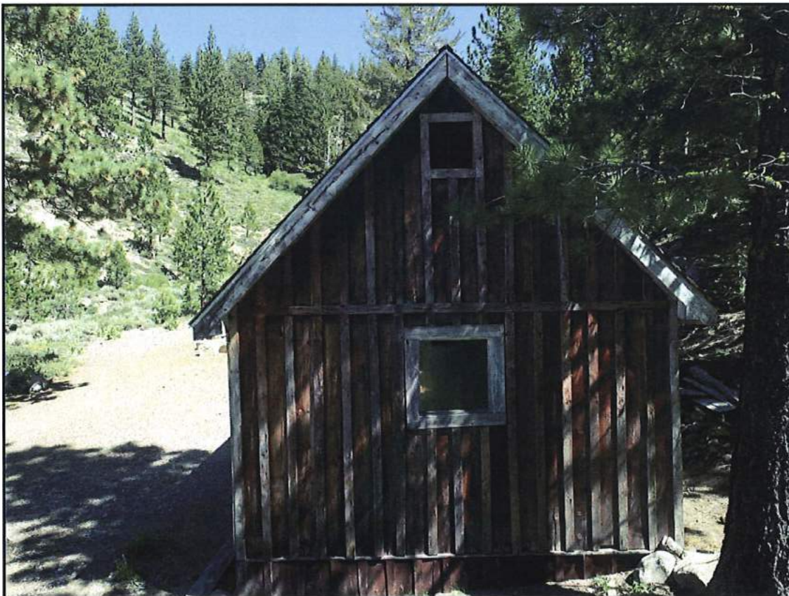
West Gable End of Building (looking northeast)
