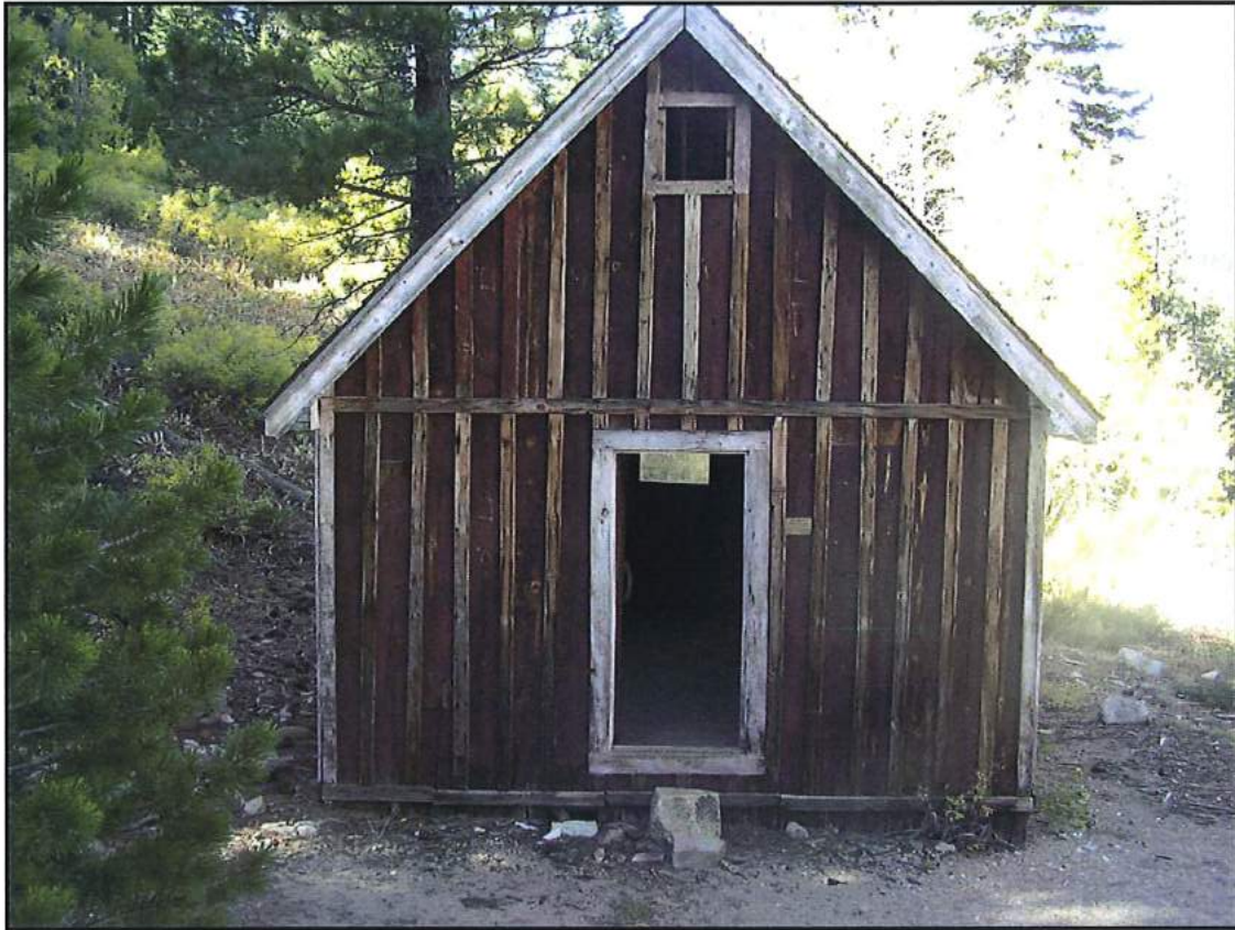
East Gable End of Building (looking southwest)
