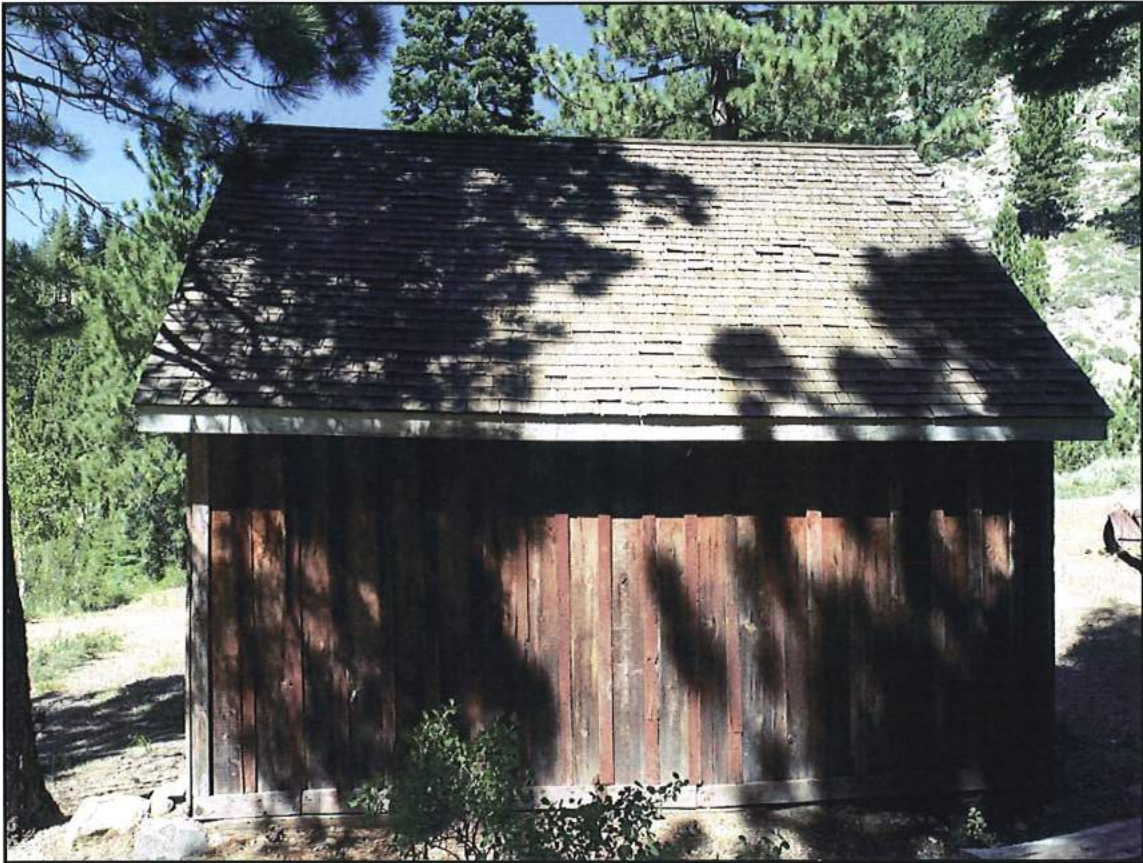
South Side of Structure (looking northeast)
