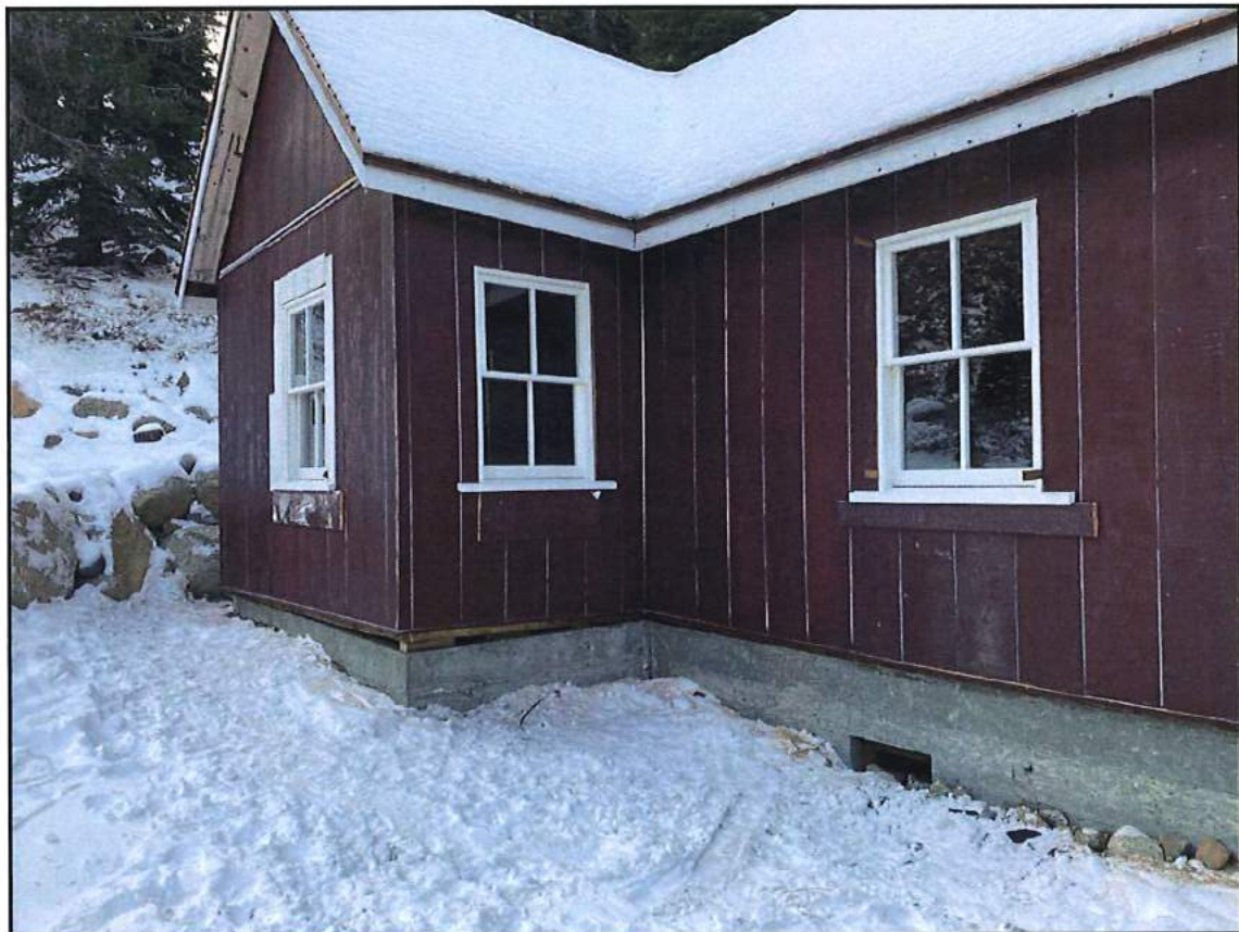
Example of rehabilitation treatment (2019 Phase 2 on Main House, without battens and plank skirting installed)
