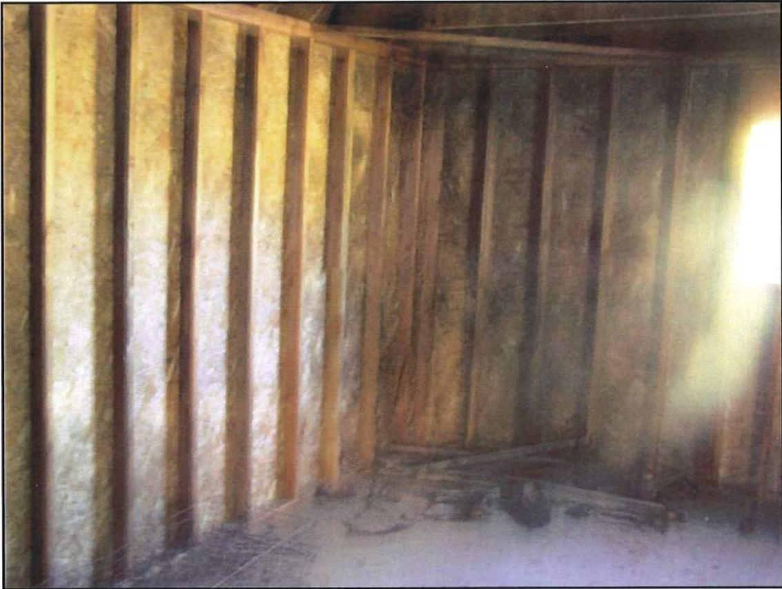
Interior of Structure (looking southwest)
