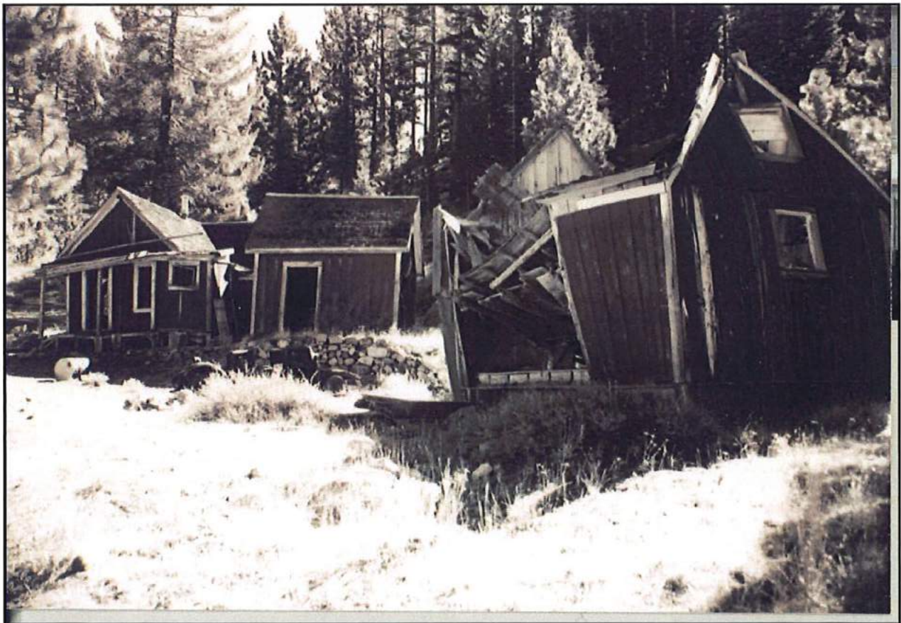
Site Picture with Bunkhouse in Foreground – early 1990's after collapse
