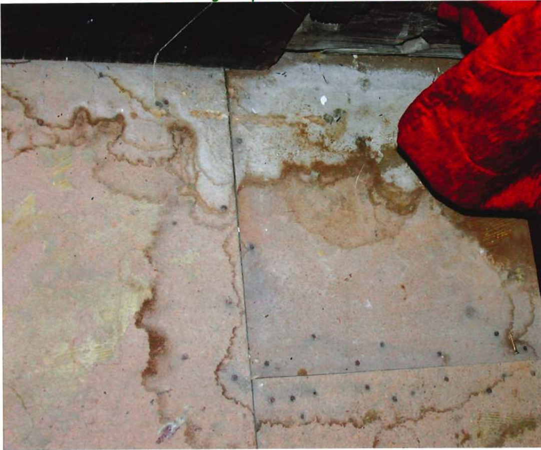
Subflooring; carpet had to be removed
