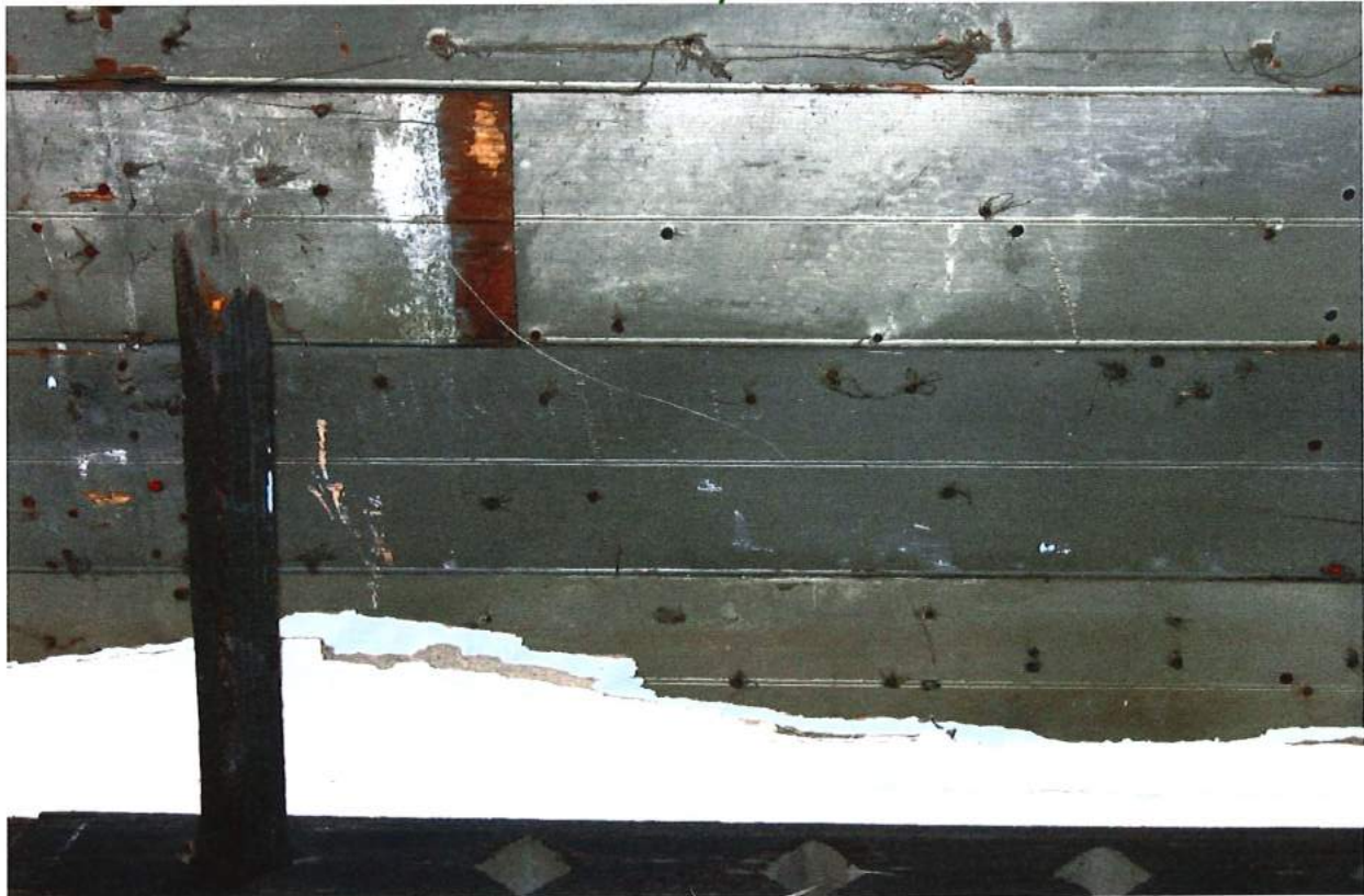
Most of the drywall cracked and fell off the ceiling exposing the original treatments. Many holes and unsecured planks
