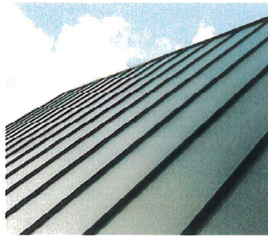
METAL ROOFING AT RESTROOMS BUILDING, TRASH ENCLOSURE AND PUMP HOUSE
