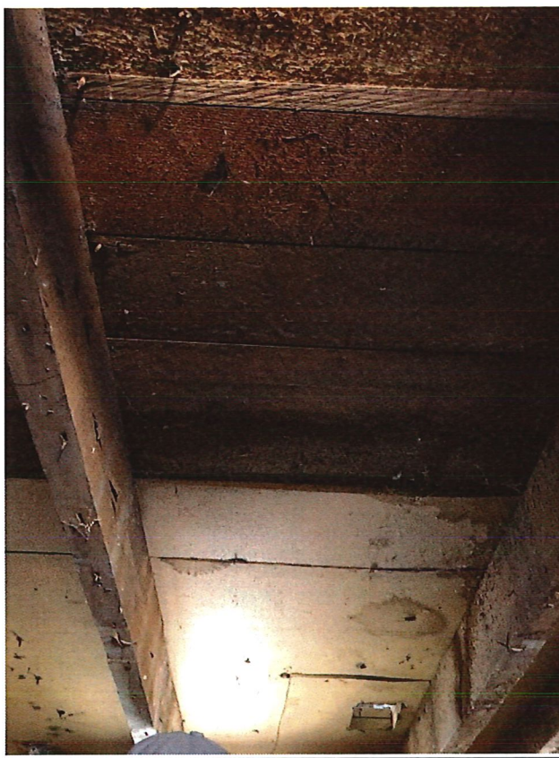
Poor hardboard subfloor in Modern Bathroom
