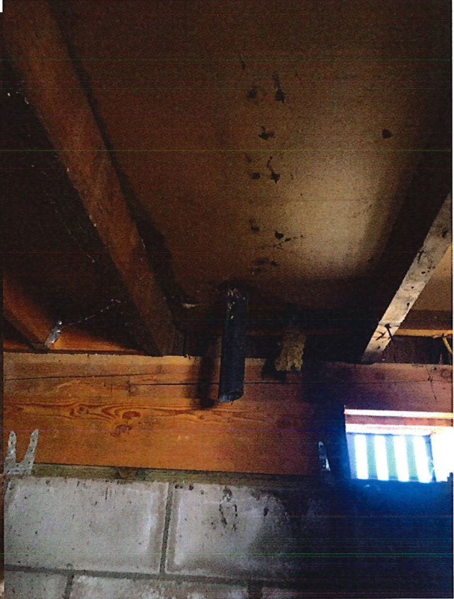
Poor hardboard subfloor in Modern Bathroom
