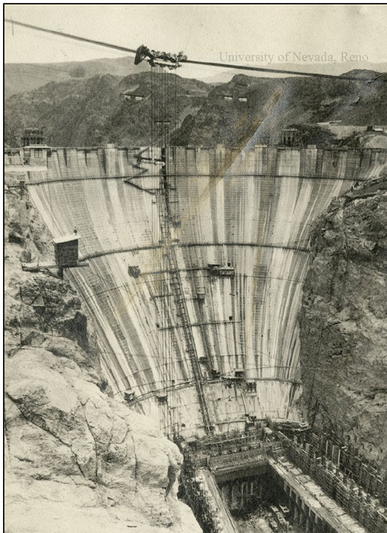
Figure 11. Hoover Dam during construction, ca. 1932. James R. Herz Collection, UNRS-P1992-01, Special Collections and University Archives Department, University of Nevada, Reno.
