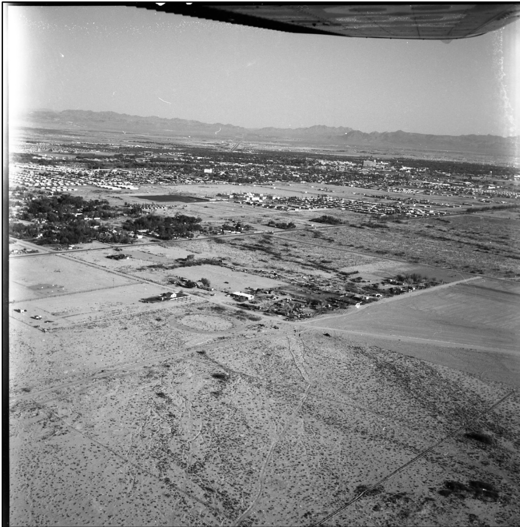
Figure 48. Aerial view of the Westside taken for purposes of urban renewal, April 11, 1963. Nevada State Museum, Las Vegas.
