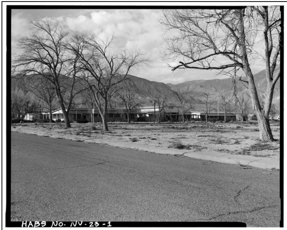
Figure 22. View to West showing Post Office/Barber Shop, Grocery Store/Meat Market, Thrift Shop and fountain - Hawthorne Naval Ammunition Depot, Babbitt Housing Area. Library of Congress, Prints & Photographs Division, HABS, HABS NV-23.
