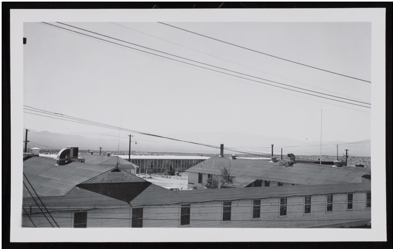
Figure 68. Buildings at Camp Williston, ca. 1940. United States Park Service Collection 0189 0024. Special Collections & Archives, University Libraries, University of Nevada, Las Vegas.
