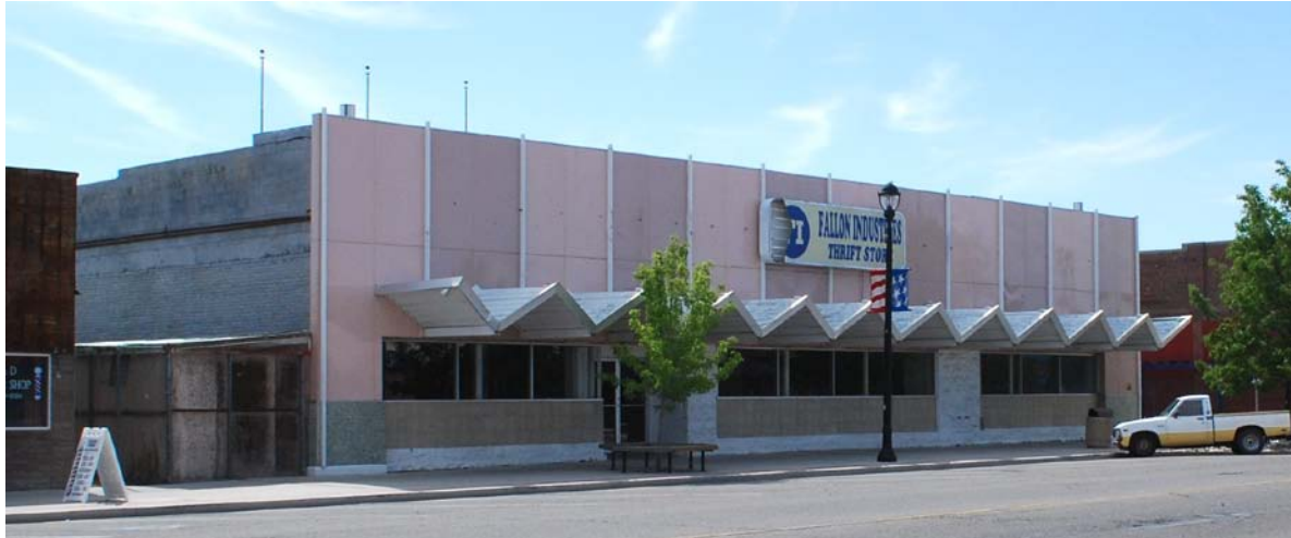
Figure 2: The I.H. Kent Store is an example of multiple Mid-Century modifications related to modernization and earthquake damage repair, October 2015.
