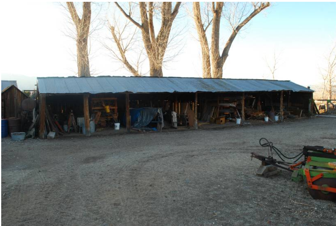
Photograph 18 – Large Loafing Shed, east façade, looking west.
