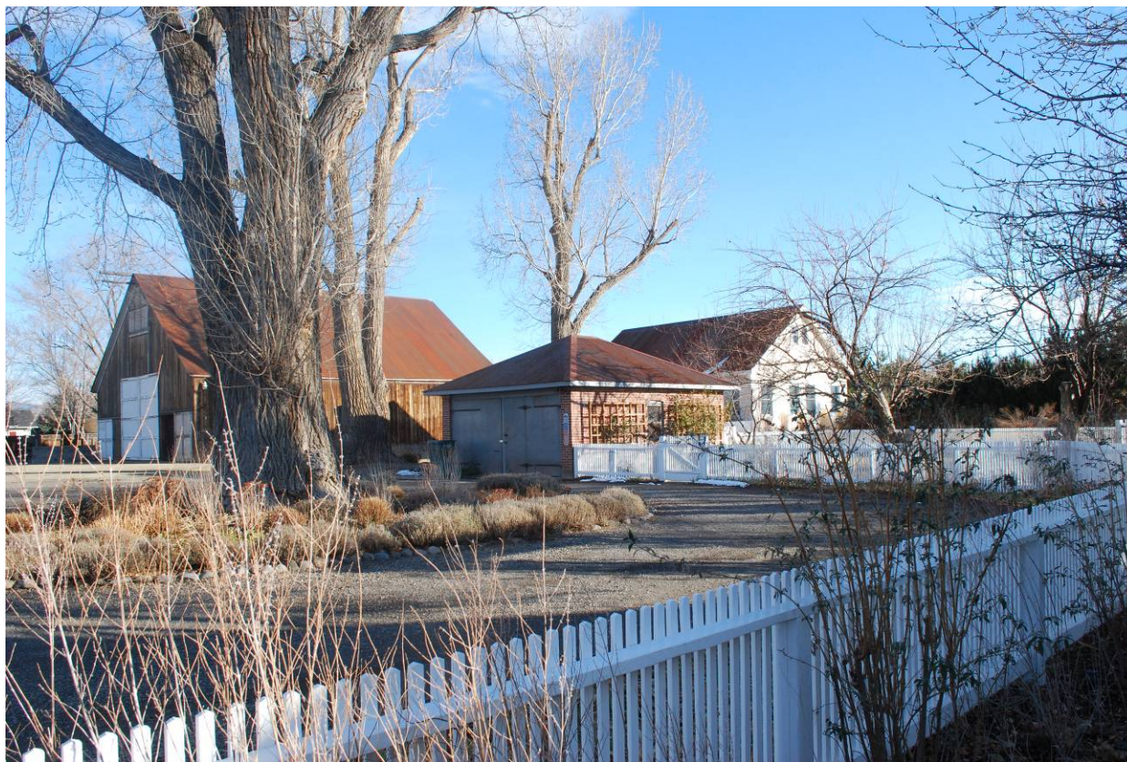
Photograph 13 – Garage (center), with Barn and Guest House in background, looking southeast.
