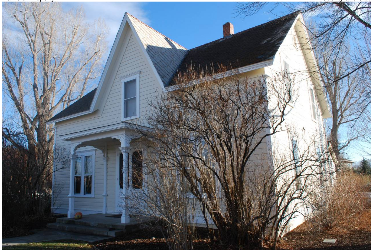
Photograph 3 – Lampe Ranch House, looking southeast.
