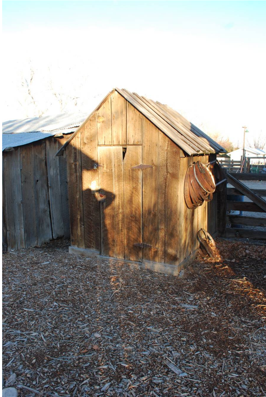
Photograph 16 – Smokehouse, west façade, looking northeast.
