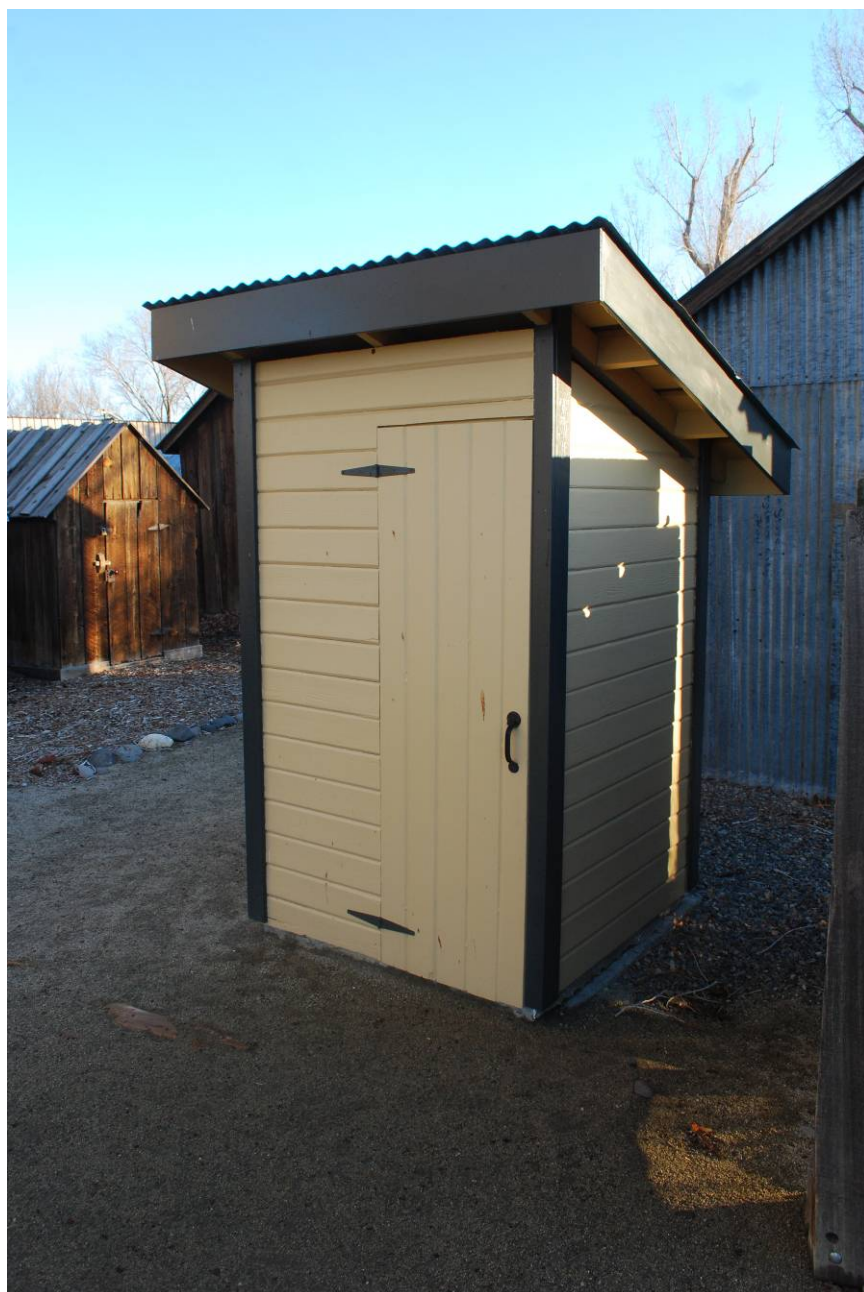
Photograph 17 – WPA Privy north façade, looking southeast.
