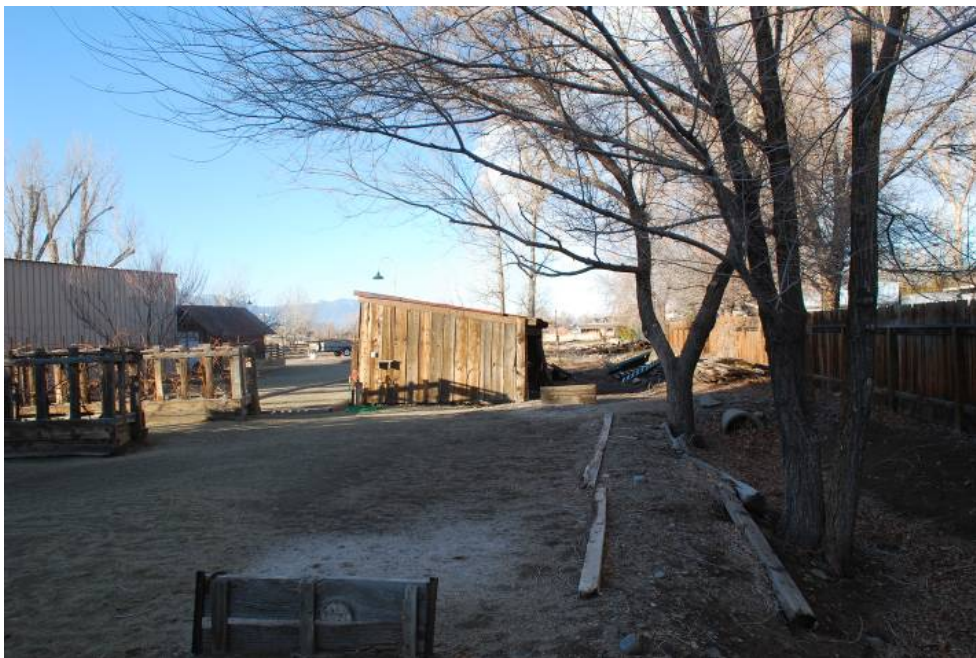
Photograph 20 – Small Loafing Shed, also showing the Hussman Company Ditch running along the fence line to the right, looking north. The Warehouse (far left) and Salvage Shed (left) are also visible.
