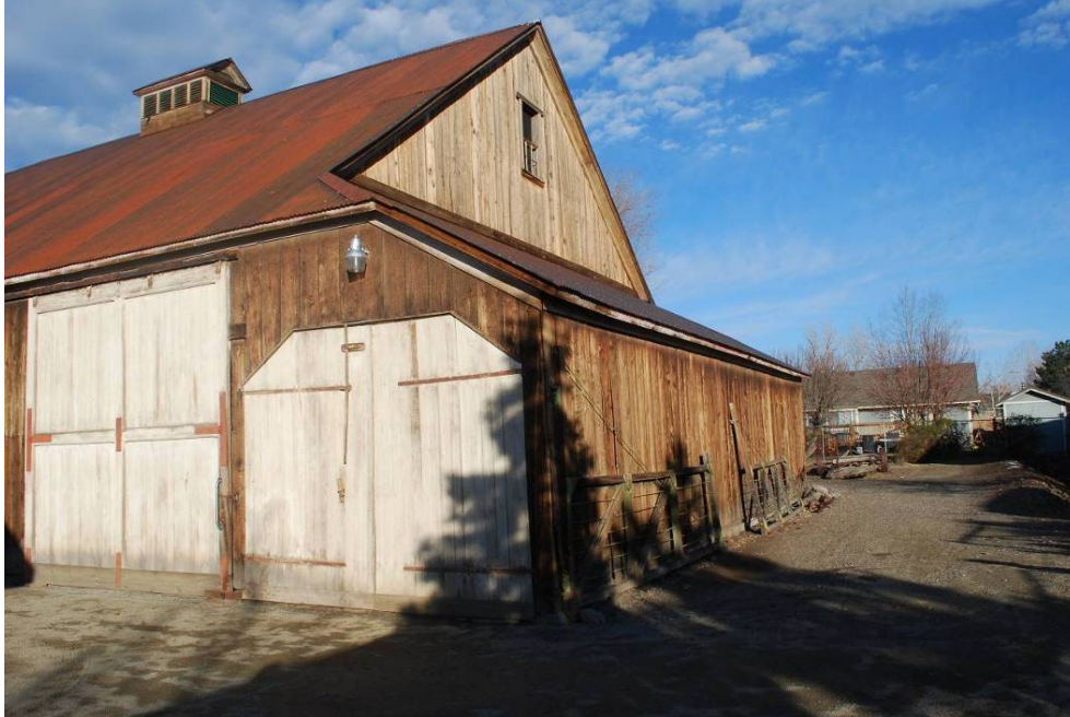
Photograph 7 – Barn, rear elevation and southwest corner, looking northeast, showing grain bin addition.
