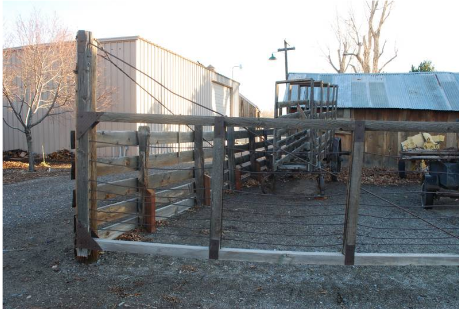
Photograph 19 – Corral and gate, looking south.
