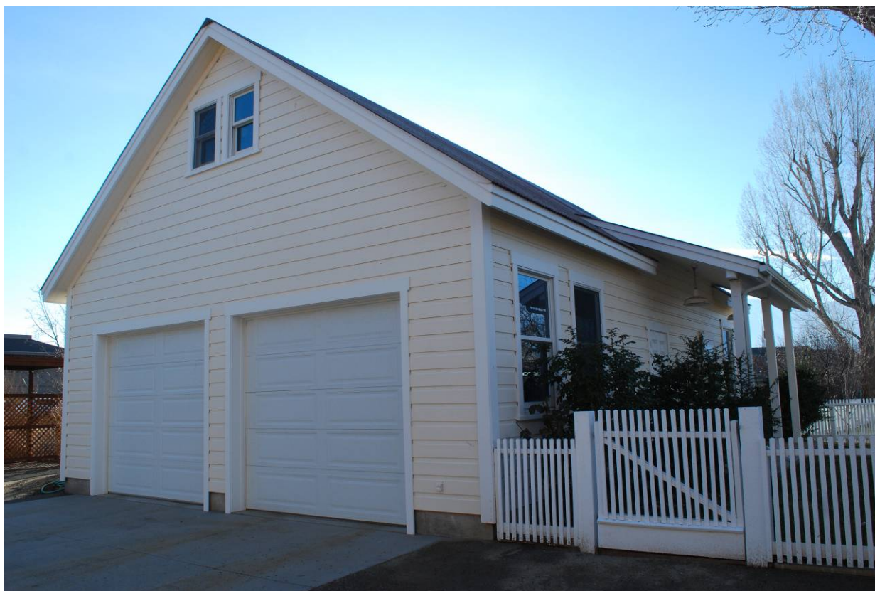
Photograph 12 – Guest House, east and north elevations, looking southwest.
